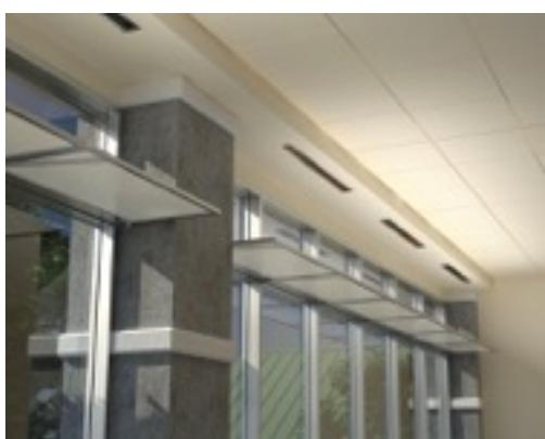
Light shelves are flat, reflective shelves that are placed in or near a window to bounce visible light up toward the ceiling. They are a low cost way to spread natural light throughout a greater portion of the building and provide a natural brightness. Light shelves also help reduce the need for daytime overhead lighting and are a great day-lighting solution.
